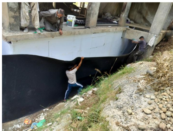
Site execution — external bitumen waterproofing coating and HDPE drain board transition at basement retaining wall
