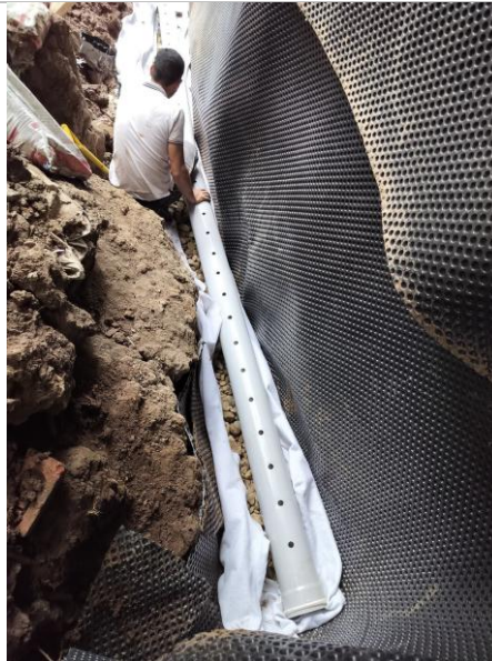
Site execution — perforated French drain pipe bedded in round rock, wrapped in geotextile, at wall footing
