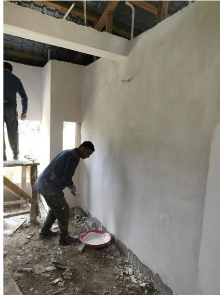
Site execution — gypsum plaster application to internal wall surface, smooth trowel finish
